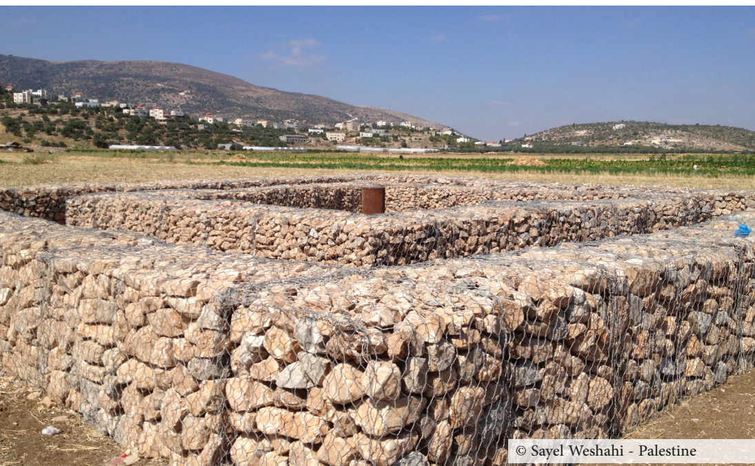
Figure 14. Filtration System - Gabions, Around an Artificial Recharge Well
