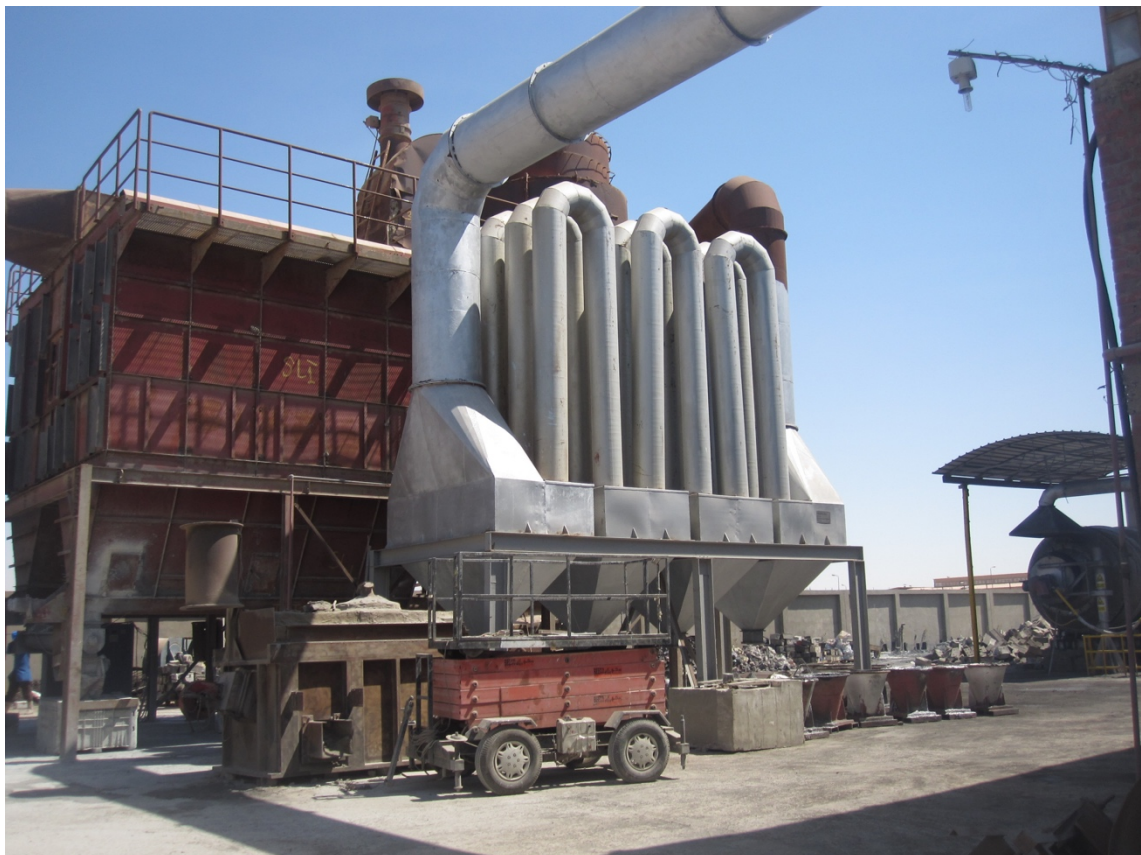
Figure 14: Bag filter at ElMotahda Facility
